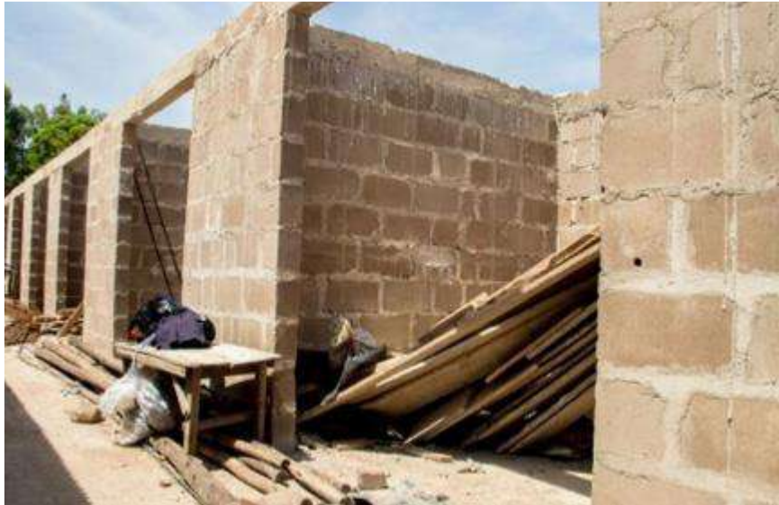
Photo 7: Mlango Mmmoja market during renovation process (Source, EfG, 2022)
